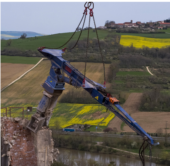
Demolition beam equipped with the AIO 601 and the CU042
